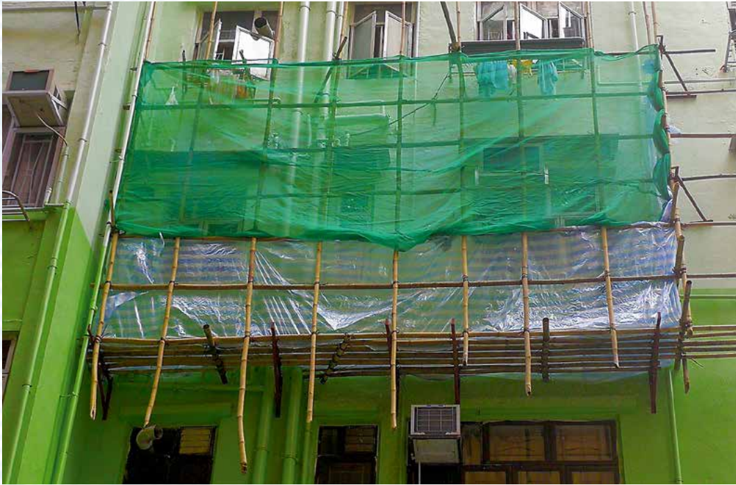
Figure 1 – Common truss-out bamboo scaffold
