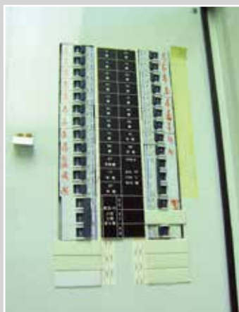
Miniature circuit breaker (commonly known as MCB) and residual current device (commonly known as RCD) equipped in electrical distribution board
