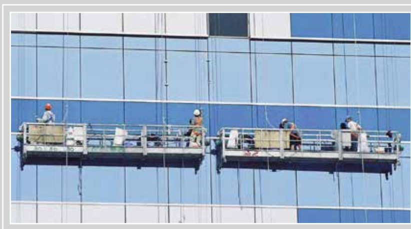
Suspended working platform undertaking curtain wall maintenance / cleaning work
