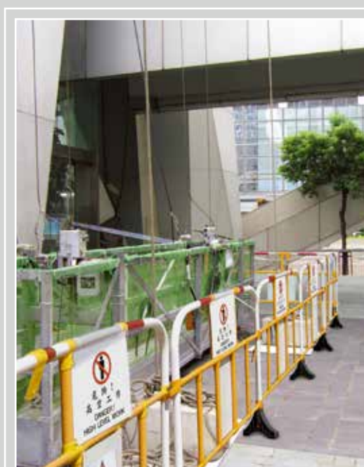
Securing the lower ends of the independent lifelines for the workers working in suspended working platform by concrete ballasts on the ground
