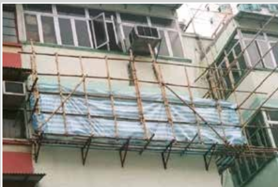
Truss-out bamboo scaffold and working platform
