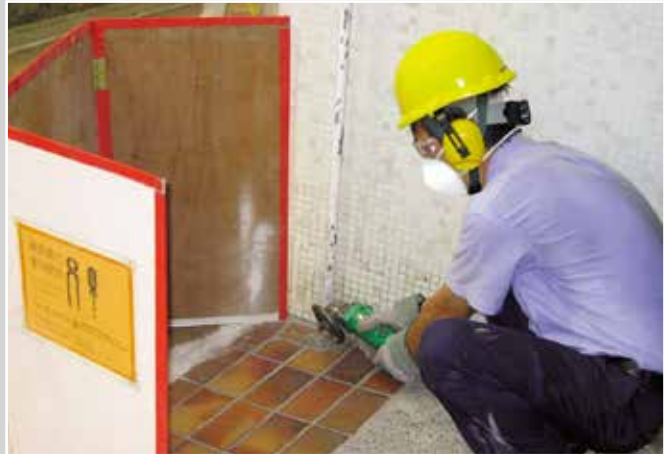
Consider other person's safety when using portable electric tools in a segregated area
