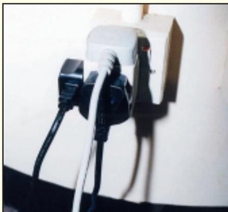
Too many plugs connected to one socket outlet is a common cause of overloading leading to electrical fire.
