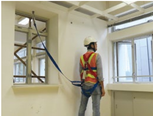
Figure 15: Full body safety harness attached to an independent anchorage
