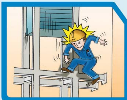
Trapped between the descending lift car and shaft structure/the counterweight inside the lift shaft
