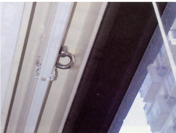
Photo 2 - an eye-bolt as the fixed anchorage
