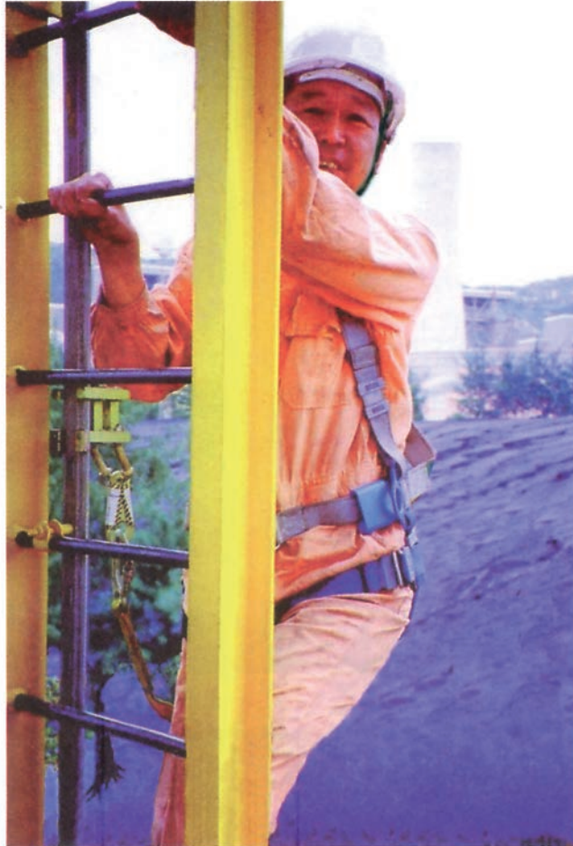
Photo 9 - guided type fall arrester on a rigid anchorage line used in power generation plant
