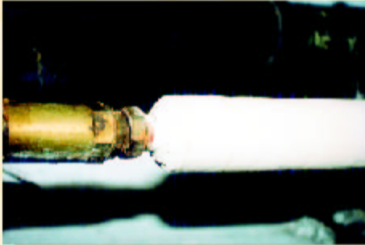
Pipe work maintenance
