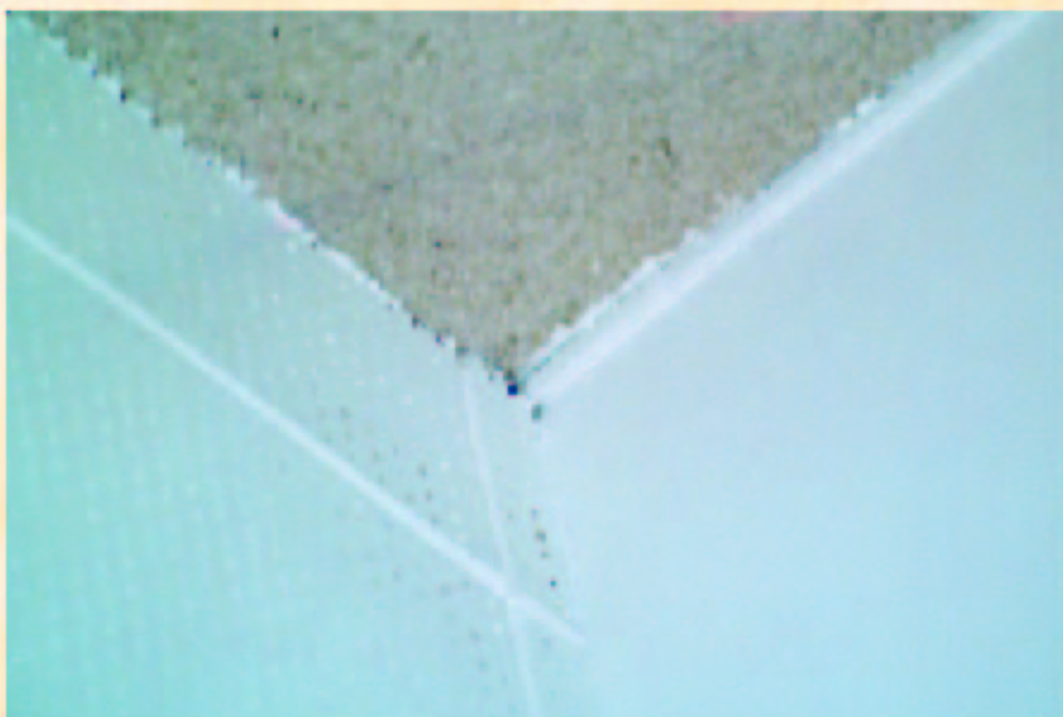
Removing acoustic plaster
