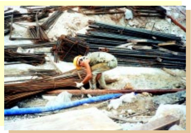
Poor manual lifting posture is a common cause of injury on a construction site.
