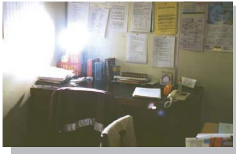
Fig. 2a Disability glare from a light fitting
