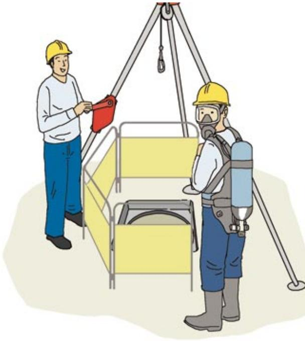
*Approved breathing apparatus should be worn in confined spaces where there are risks of the worker being overcome by hazardous gases.*
