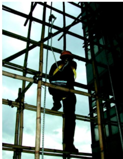
defects on the safety belt, any suitable anchorage, independent lifeline and fall arresting device, and whether the standard is met or not.
