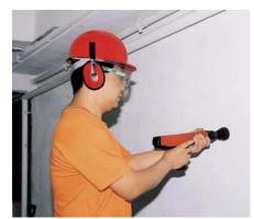
noise, such as piling work, earmuffs and ear plugs may be used together to provide better noise reduction.
