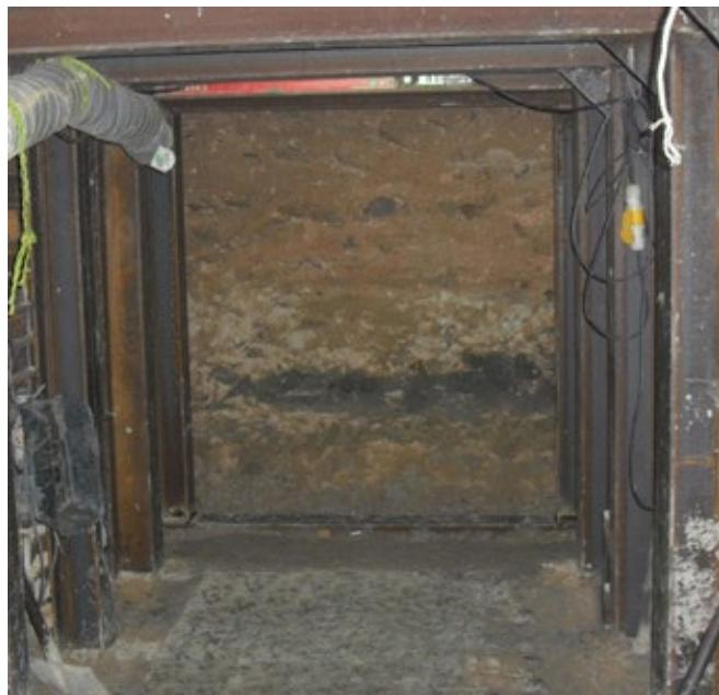
Photo 2 - A tunnel constructed by heading method
