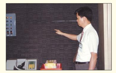
The walls of the room housing notecounting machines can be dressed with noise absorbing material to reduce reverberant noise.
