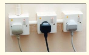
For each electrical appliance, particularly for one with high rating capacity, there should be one independent socket outlet.
