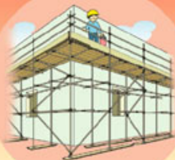
Double row scaffold and working platform
