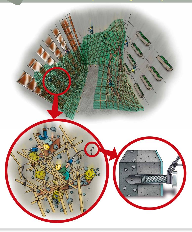
Renovation works were being undertaken on the external walls surrounding an internal courtyard of a building complex. To facilitate the works, four panels of double-row bamboo scaffolds were erected on walls from 2/F up to the roof.
