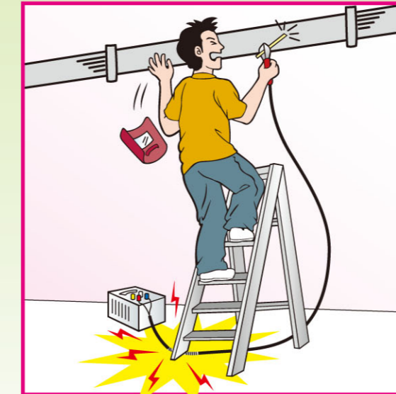
Pay particular attention to trailing electric wires and avoid using ladder when engaging in electric welding
