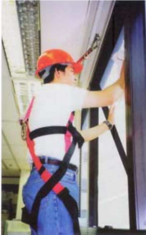
Photo 1 - windows cleaning work using full-body harness and fixed anchorage
