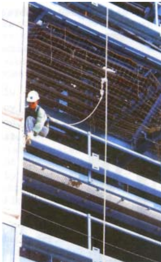
Photo 3 - external window panel installation work using rope chuck and vertical independent lifeline
