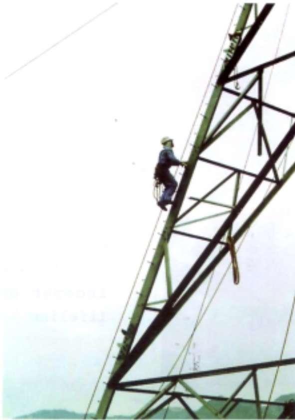
Photo 6 - electrical t o w e r assembling work using guide rope, rope grab and rope adjuster
