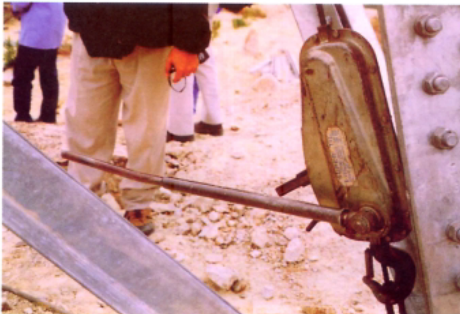
Photo 7 - the rope tension adjuster used in tensioning the guide rope
