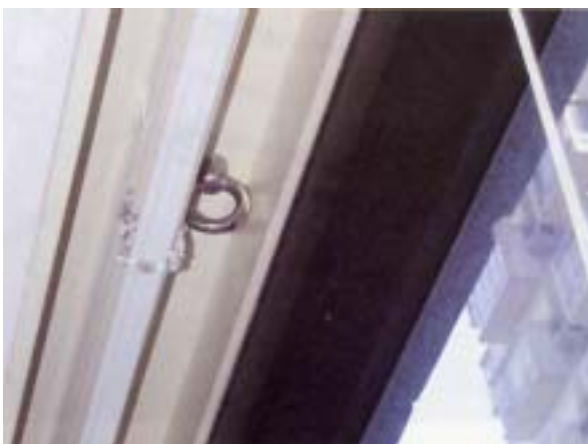
Photo 2 - an eye-bolt as the fixed anchorage
