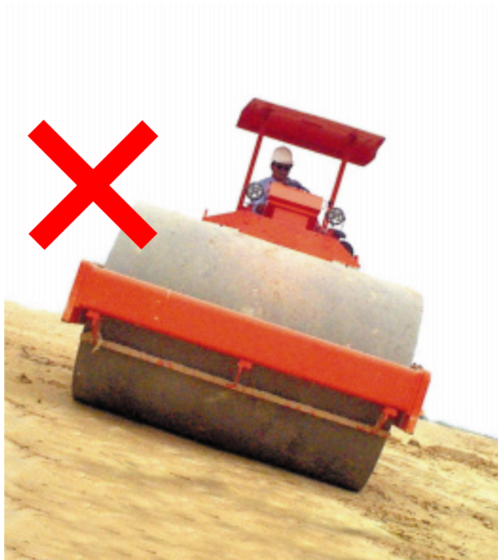
Fig . 5 When working on slope, avoid sidehill travel
