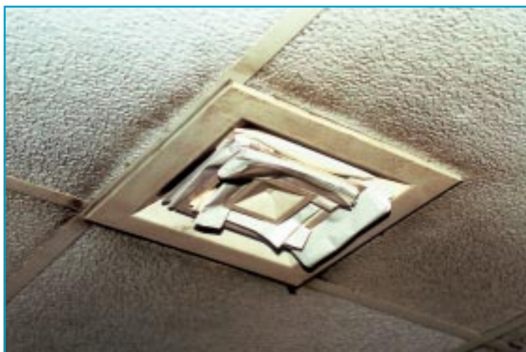
Unbalanced ventilation may disturb the room temperature and air distribution. Tampering with an air outlet may further upset the balance
