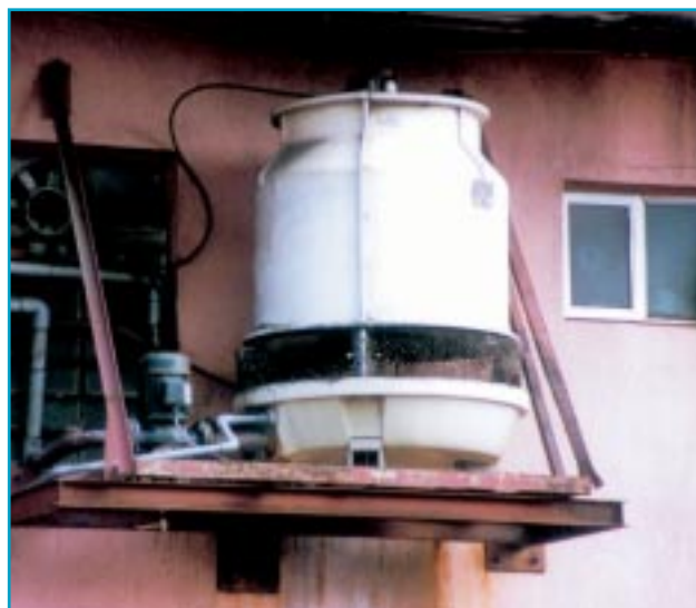
A water cooling tower
