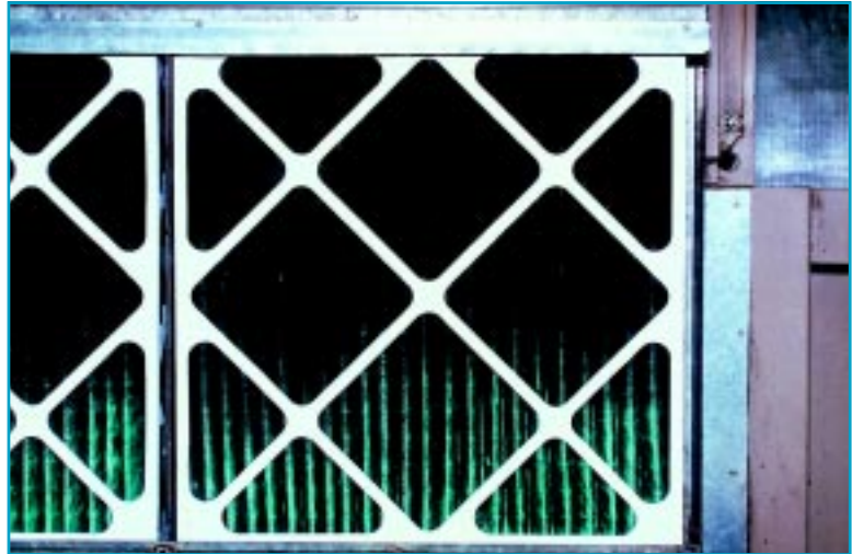
Mould growth on dirty filters
