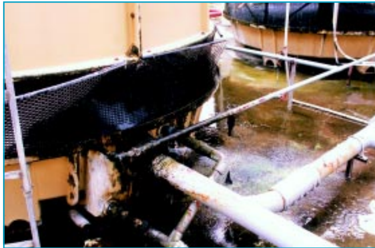
Poor maintenance may create an ideal breeding ground for micro-organisms.
