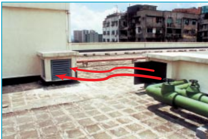
Intake points should not be too close to exhausts
