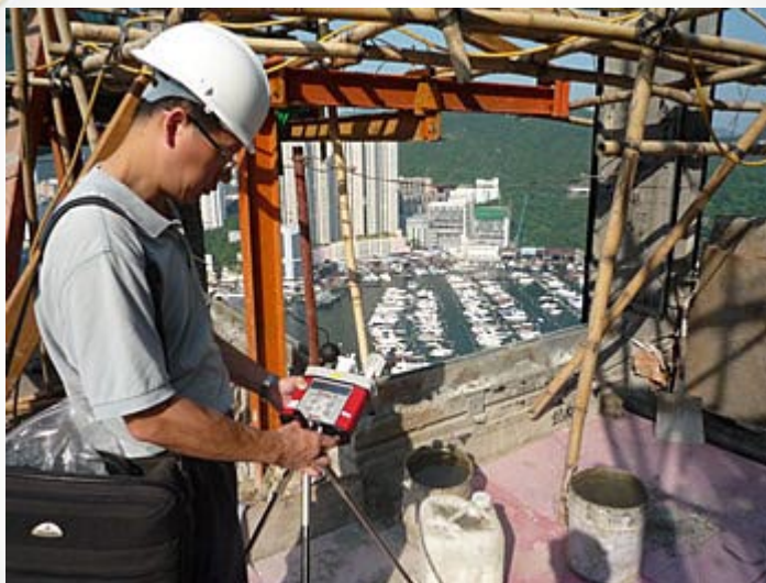
An Occupational Hygienist assessing the risk of heat stress at a construction site
