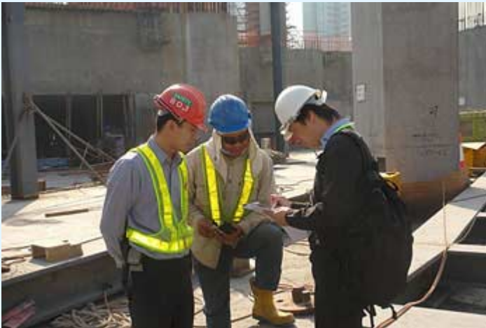
An Occupational Safety Officer conducting inspection at a construction site.
