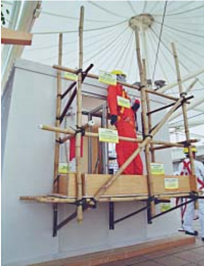
Truss-out scaffold work safety exhibition.
