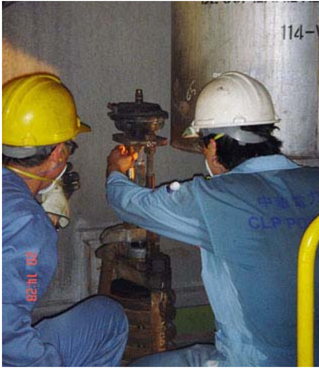
Joint inspection of a boiler by a surveyor and an appointed inspector.
