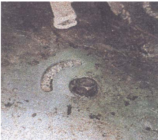
Photo 1.3 Hole for relief valve was fitted with bolt and nut
