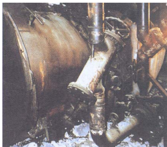
Photo 22.4 Whole boiler room was badly damaged
