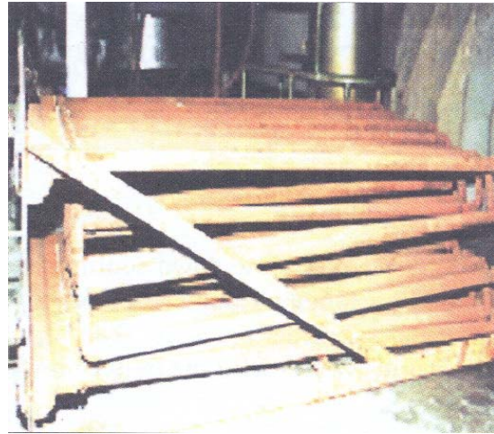
Photo 24.2 Cooling coil inside the blow-down tank
