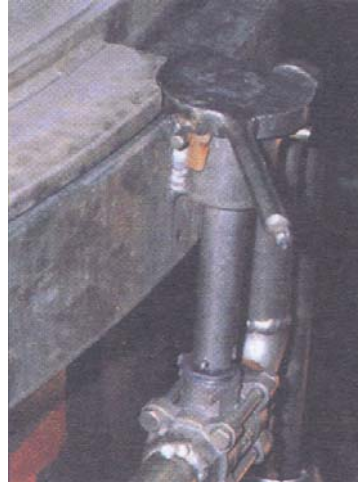
Photo 6.2 Interlock exhaust valve in its closed position
