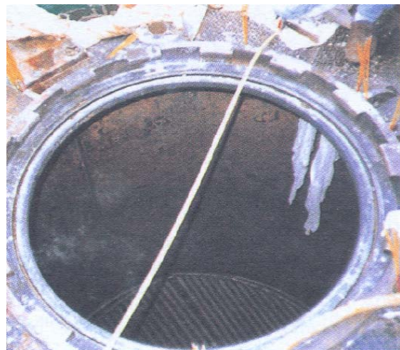
Photo 11.2 Close-up of the interior of the steam kler
