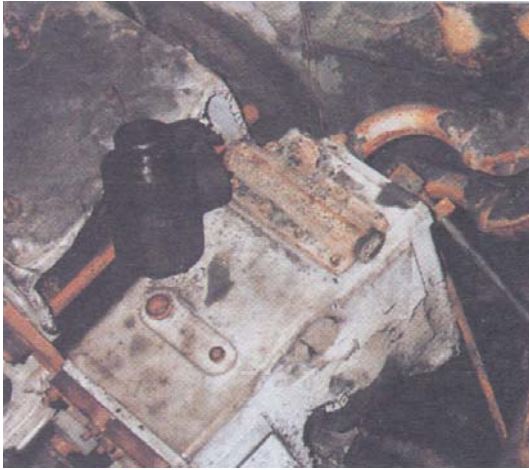
Photo 4.1 Damaged burner gear
