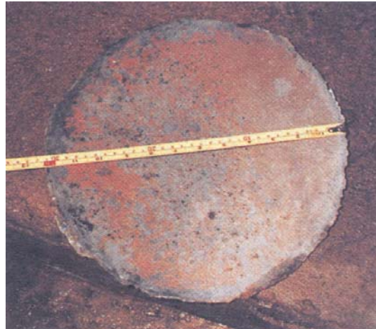
Photo 7.4 Detached end plate of the steam manifold
