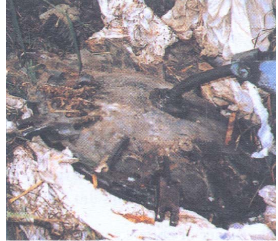
Photo 11.4 The bent lifting spindle of the kler cover
