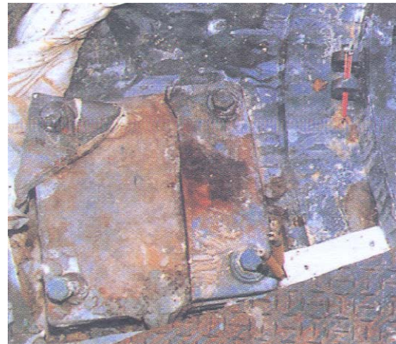
Photo 11.6 Full-width crack on flat base of the cast-iron pedestal column
