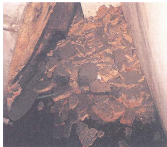
Photo 15.4 Blown off rear end cover with collapsed refractory
