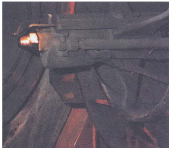
Photo 23.2 The leaky burner tips and air diffuser with carbon deposits
