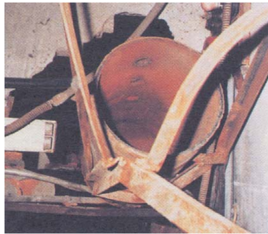
Photo 7.2 End View of the steam manifold
