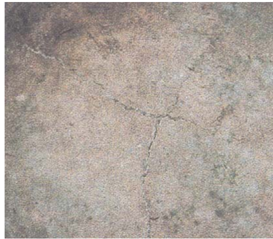
Photo 1.2 Crack on the bottom
