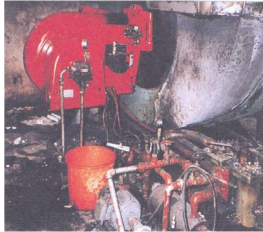
Photo 5.2 Damage to boiler and fuel oil system
