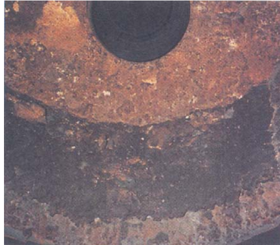
Photo 23.4 Damaged furnace refractory
