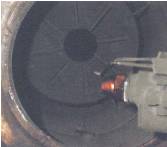
Photo 23.3 Air diffuser and wet burner tip
