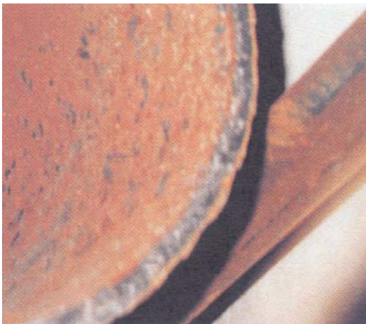
Photo 7.3 Close-up view to show the failed edge of the steam manifold
