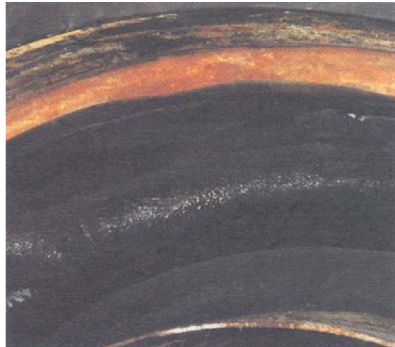
Photo 22.2 Through crack on the shell of the thermal oil heater
