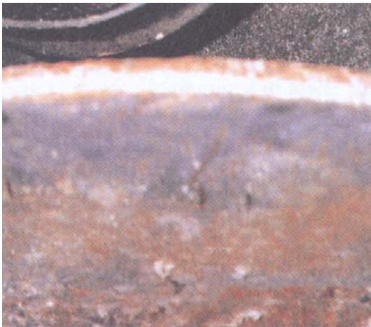
Photo 8.3 View of the edge of the steam manifold from bottom
