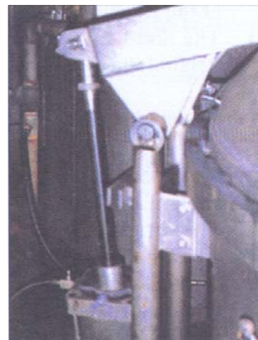
Photo 6.8 Pneumatic actuator for lifting the kier cover
