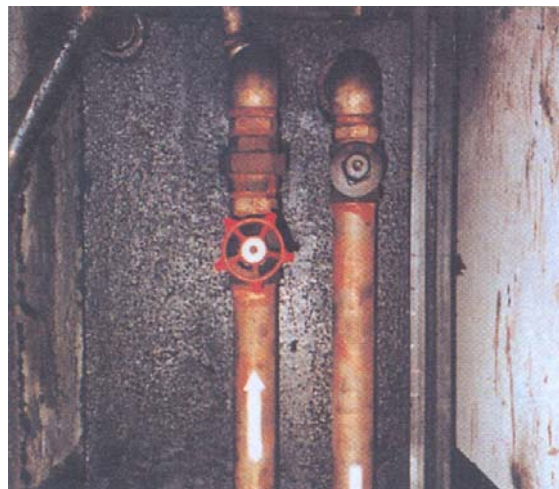
Photo 23.6 Fuel oil tank with supply & return fuel pipes
