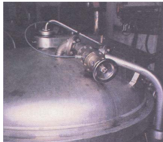
Photo 6.5 Pneumatic overflow valve at the kier cover
