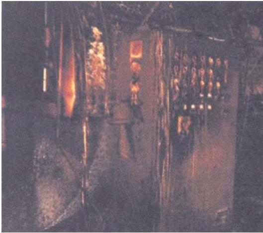
Photo 5.1 Damage to boiler
