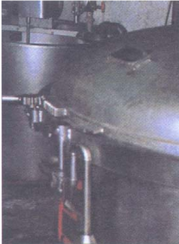
Photo 6.1 Kier cover is being unlocked
