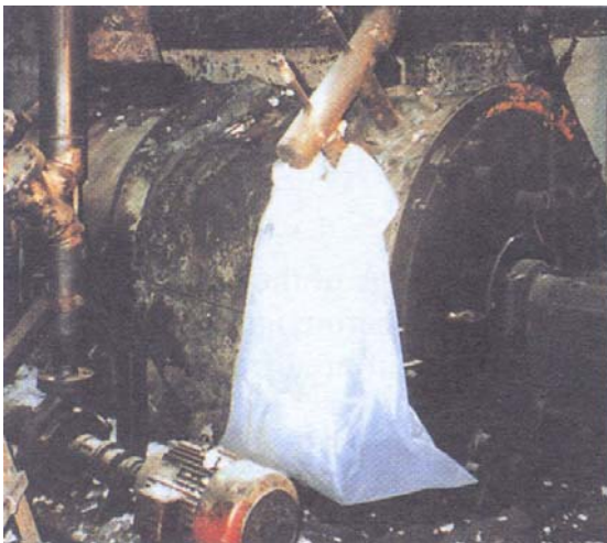
Photo 22.3 No save-all was fitted underneath the circulating pump
