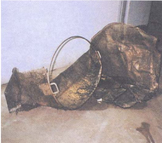
Photo 3.1 Damaged strainer of the cauldron
