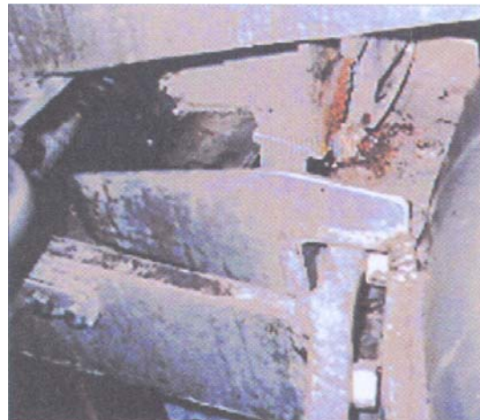
Photo 13.6 Broken level indicator, broken guide-pin and its bracket
