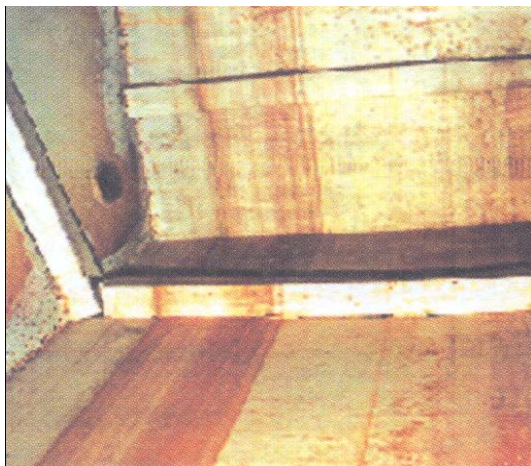
Photo 24.5 Inadequate stiffeners were installed inside the poorly constructed blow-down tank
