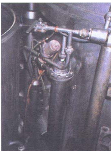
Photo 6.6 Manual overflow valve
