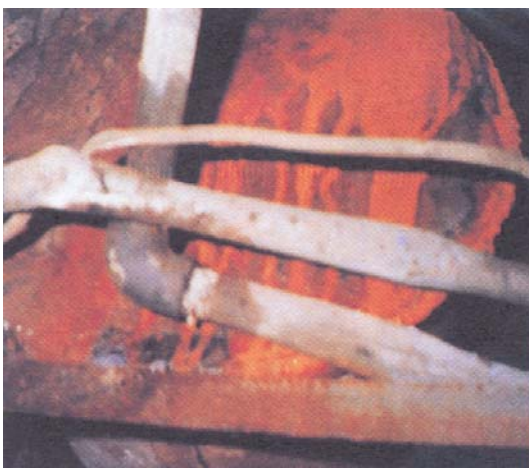
Photo 7.5 Weld on the other side of the steam manifold
