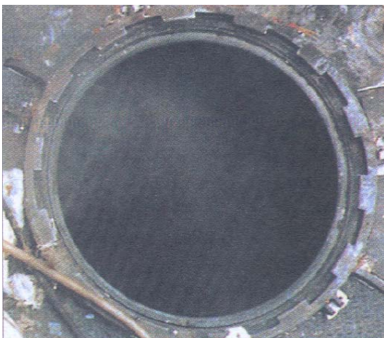
Photo 11.5 5 of the 7 cover locking bolts were sheared away
