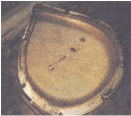
Photo 3.3 Damaged lid with fittings
