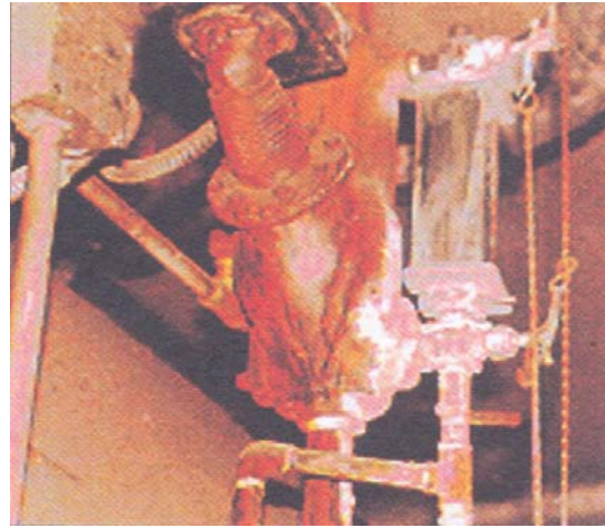
Photo 19.2 White deposits were lodged on the water level gauge glass
