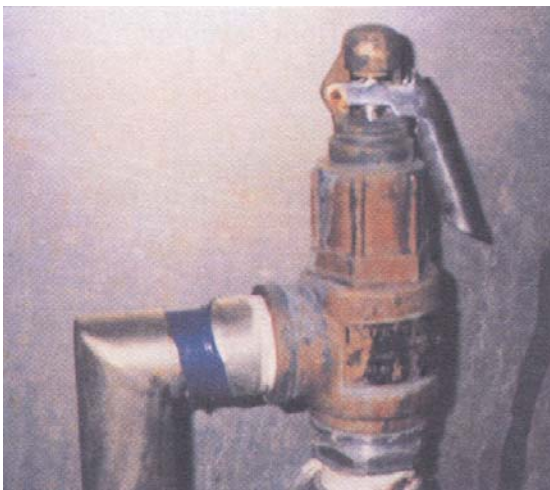
Photo 6.4 Seal for safety valve was missing
