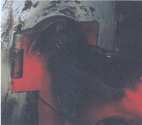
Photo 23.1 The damaged and blacken burner unit
