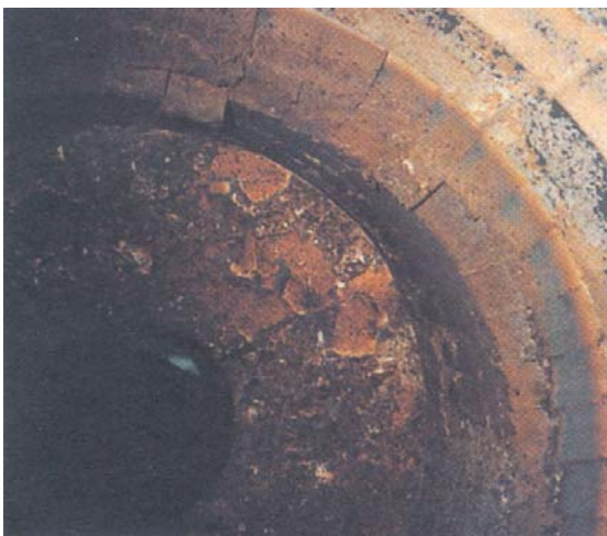
Photo 23.5 Built-up slag at combustion crown
