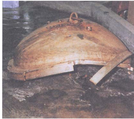
Photo 3.4 Damaged lid with fittings removed
