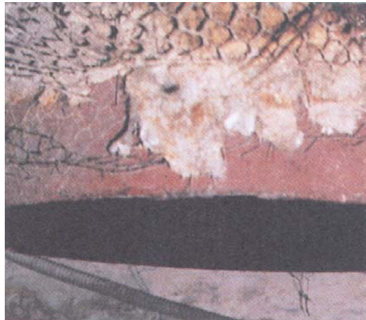
Photo 8.4 View of the edge of the steam manifold viewing from top
