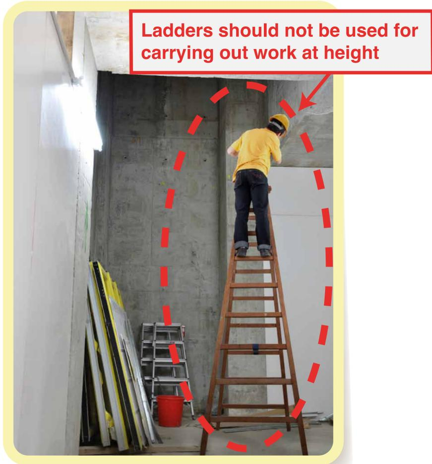
Ladders should not be used for carrying out work at height
