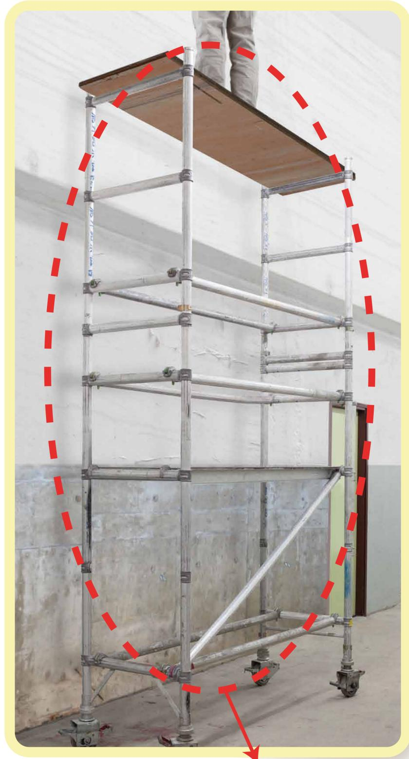
No guard-rails, toe-boards, outriggers or access and egress are provided on the working platform
