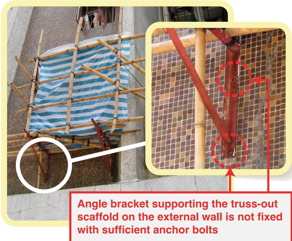
Angle bracket supporting the truss-out scaffold on the external wall is not fixed with sufficient anchor bolts
