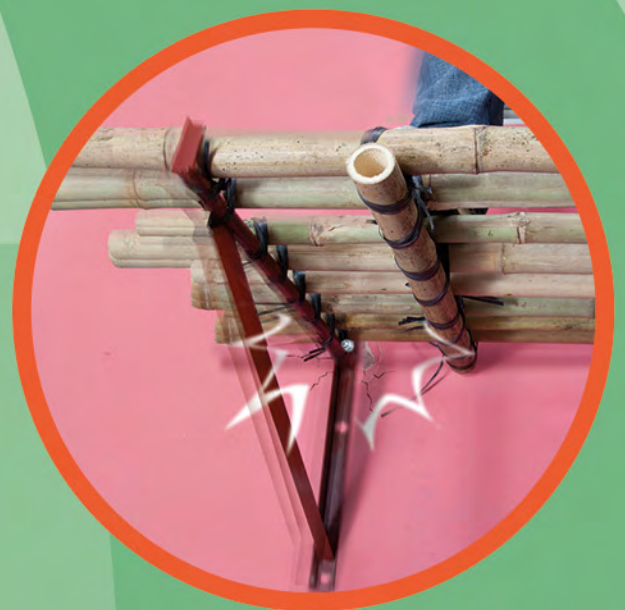
The angle bracket was fixed by one bolt only
