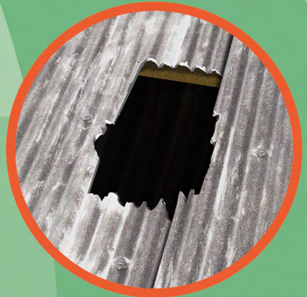
The roof was fragile
