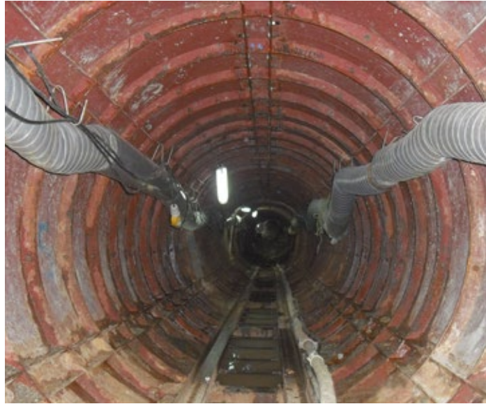
Photo 1 - A tunnel constructed by use of prefabricated segments
