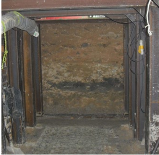
Photo 2 - A tunnel constructed by heading method
